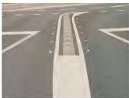
Part of the roadway is raised creating a danger for a PTW (Source: IBZH, NL)
