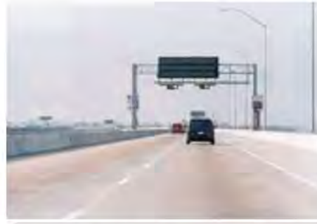
Examples of Jersey roadside barrier (source: ITC, Bulgaria)
