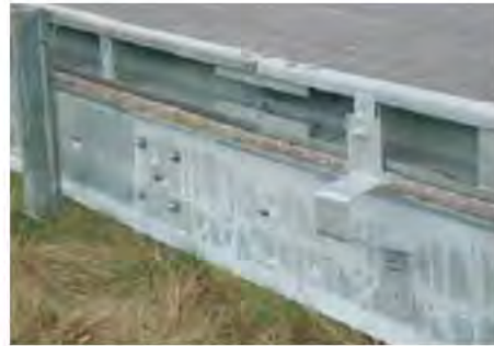
Example of PTW-friendly safety barrier: riders are protected from the support posts (Source: http://www.fema.ridersrights.org and Internet)
