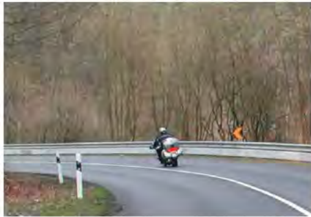
Example of PTW-friendly safety barrier: riders are protected from the support posts (Source: http://www.fema.ridersrights.org and Internet)
