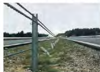
Example of a cable barrier ( http://www.fema.ridersrights.org )
