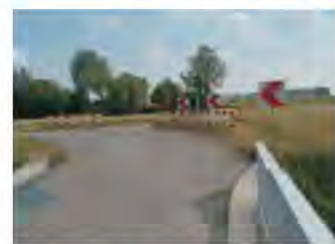
Warning sign on the outer curve may present hazard to PTW (H.Monderman, NL)
